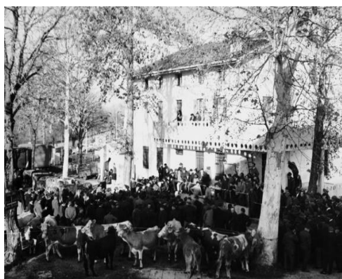
Figure 24 Historical picture of the Delle Acque Place
